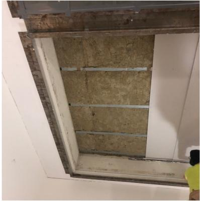
Figure B2.2: Unmounting of the installation. Shows rails, mineral wool and 2 layers of gypsum board.
