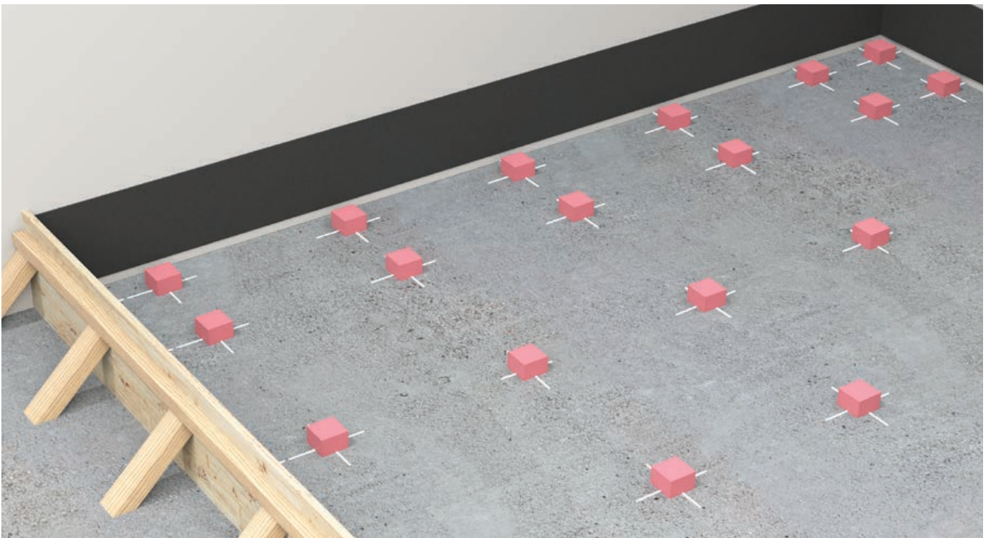
Image B-2: Use glue to fixate the position of the elastic pads.
