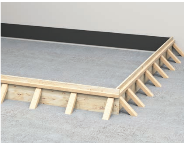
Image A-2: Formwork
