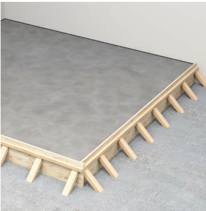
Image E-1: Finished concrete slab.
